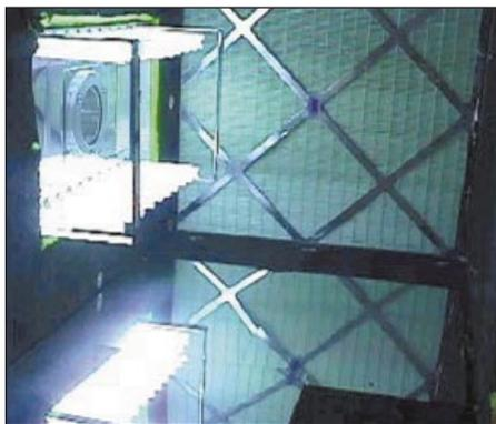
PHOTO A. UVGI array used for air disinfection. Note the specular reflective surfaces. Photo courtesy of Lumalier Inc., Memphis.
